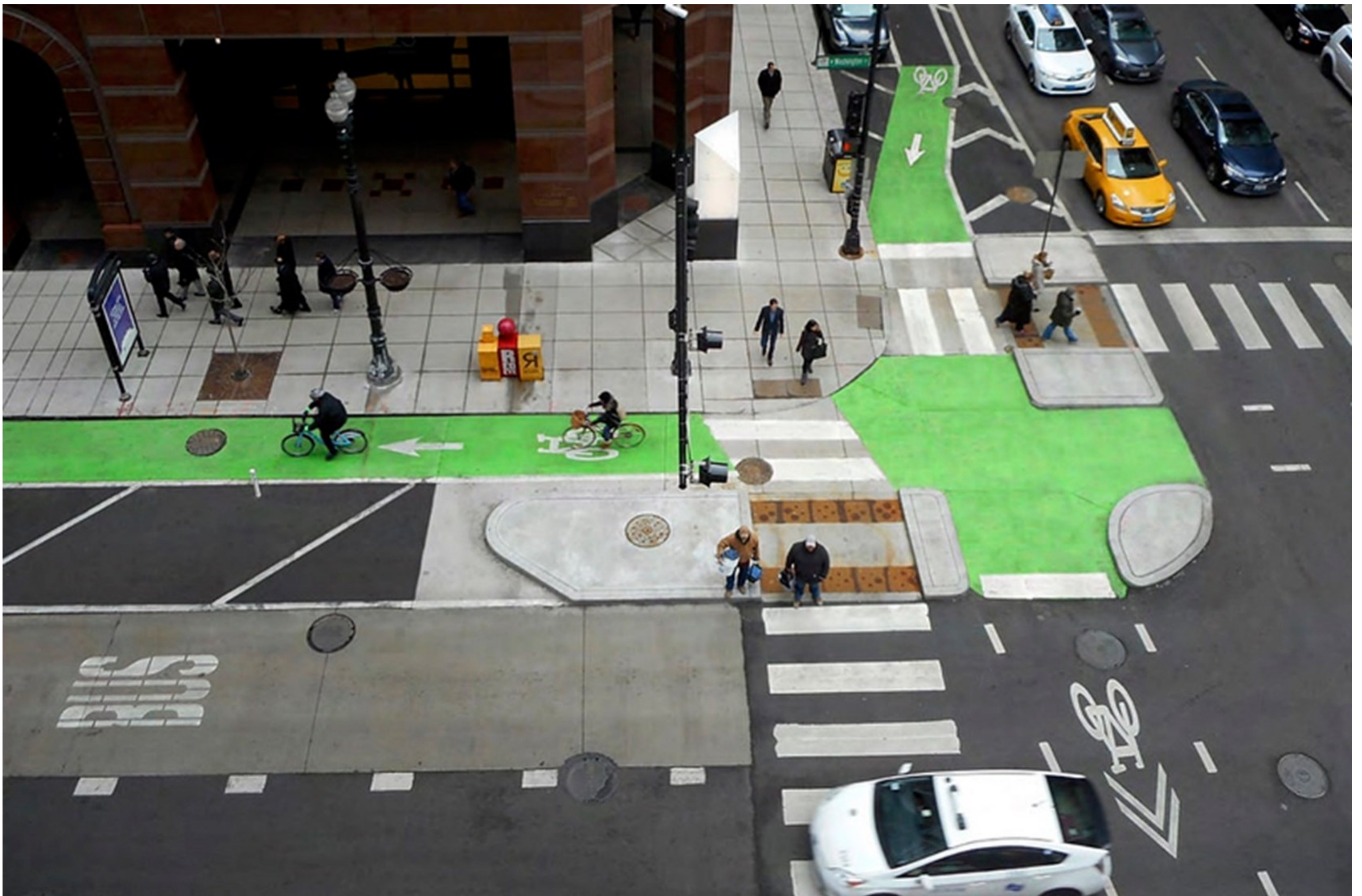
EXAMPLE OF PROTECTED INTERSECTION DESIGN - CHICAGO
